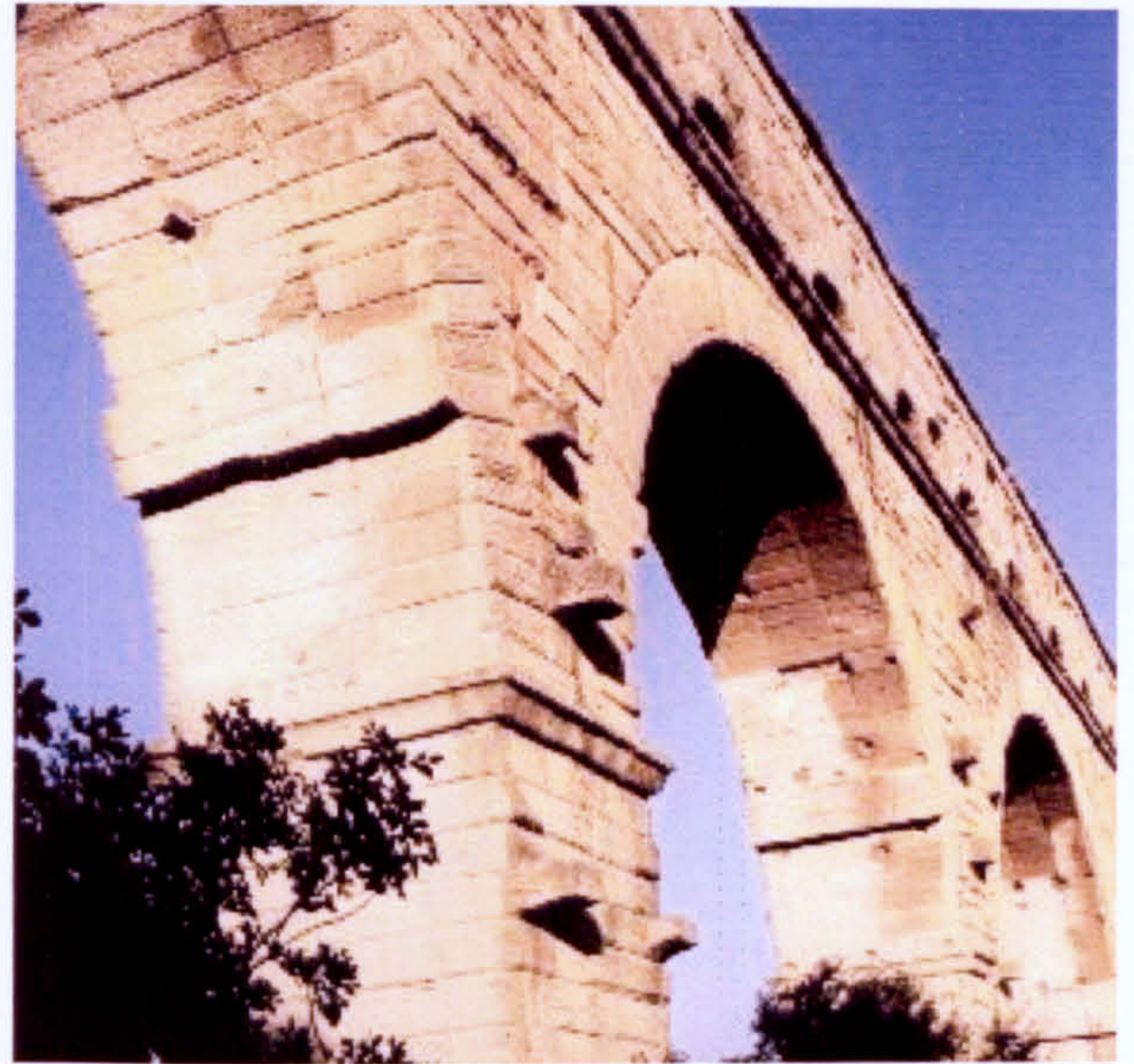
Pont du Gard, Nimes, France, example of Roman construction using masonry and lime Pozzolana concrete.
