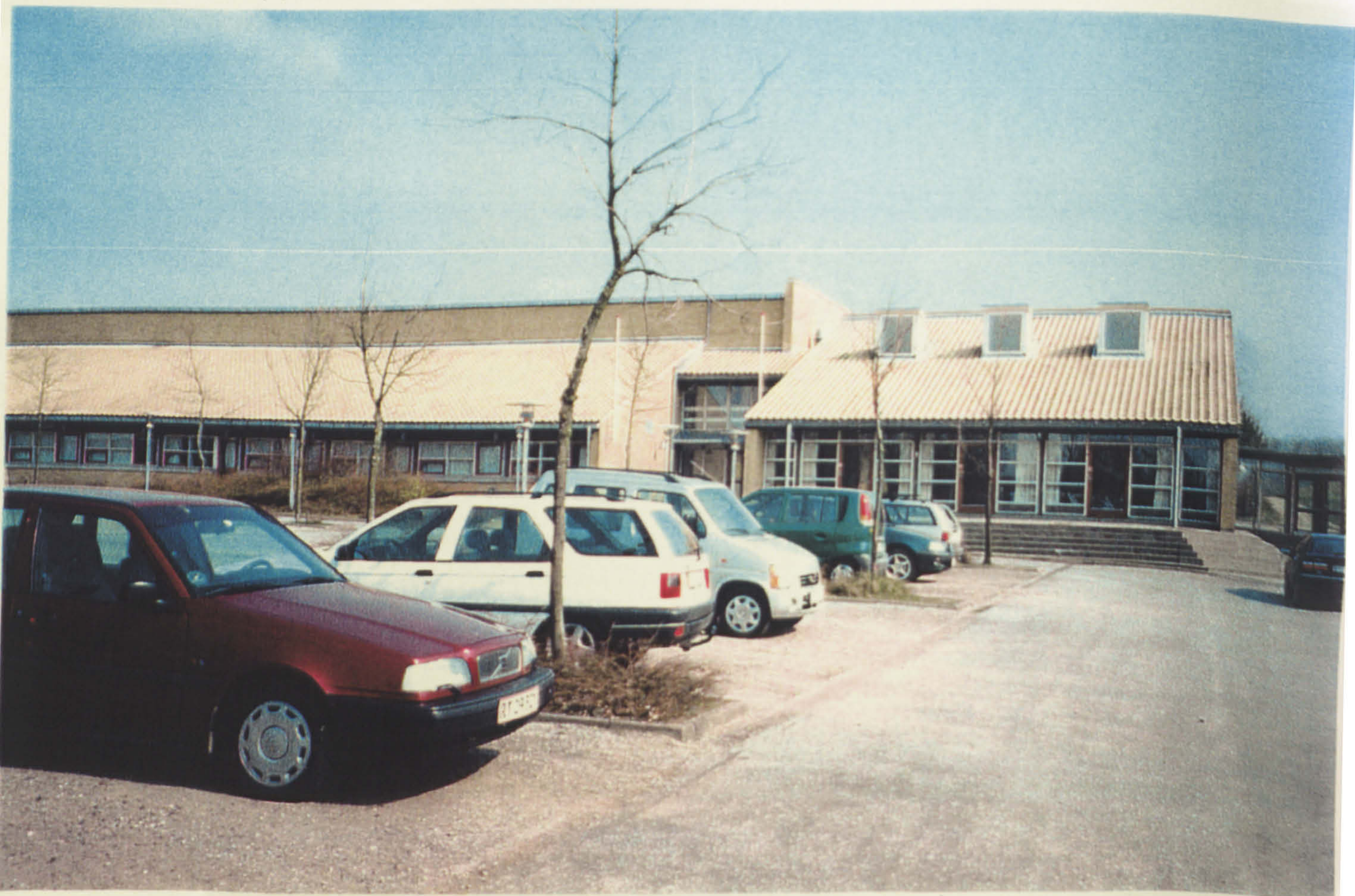
(c) Modern single-storey school building
