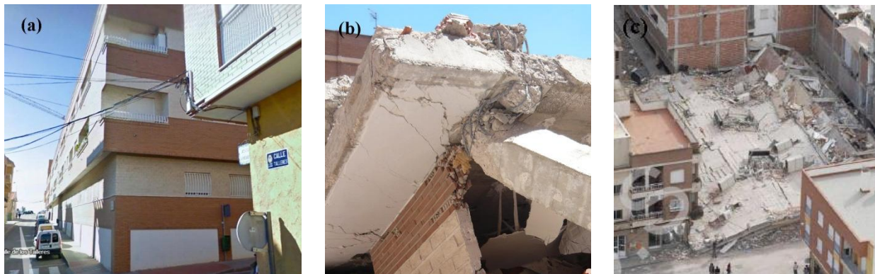
Figure 10. The only building collapsed due to the Lorca earthquake, before (Google Street View) (a) and after the event (b), (c). Photograph (c) adapted from Regalado (2011).
