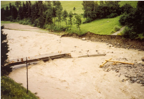
Fig. 12 Bridge destroyed across the Passer/Passirio river soon after the flood event in July 18th, 1987. The bridge was occluded with woody material and was destroyed after the outbreak of the river on the left side . The figure shows only the driftwood at the bridge that remained after the event
