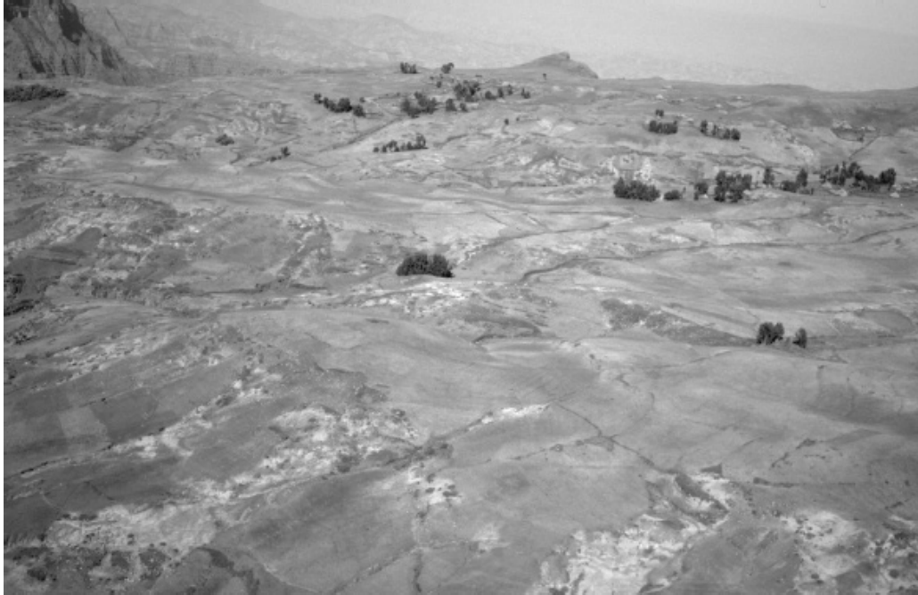
Figure 18-2: Soil degradation is widespread even within the SMNP, as seen here for the Gich area. This is a major threat to the survival of the local land users (Photo Hans Hurni, October 1994)
