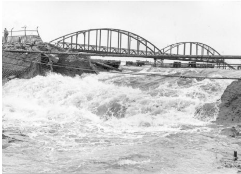
Figure 1. Broken dike after the storm surge in Hamburg in February 1962. Source: Hamburger Morgenpost, reprinted with permission.
