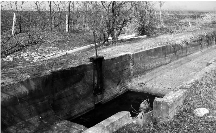
Fig. 1 Widespread broken water distribution devices hinder effective water management in the Chuy Valley. (Photo by Daniel Maselli, Sokuluk Rayon, 21 March 2003)
