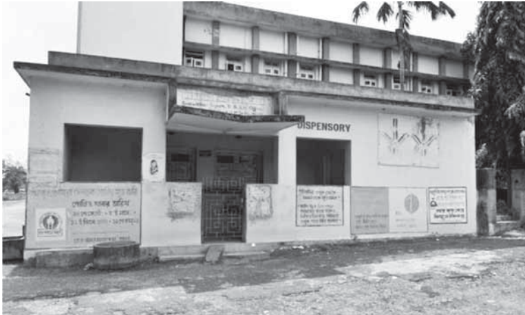
Fig.4. 28 Glimpse of Government Hospital at Digha
