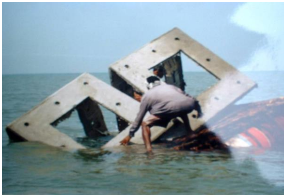
Modules sliding down to reef site (Thikkody, Kozhikode)
