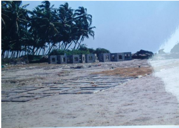
Fabrication of reef modules
