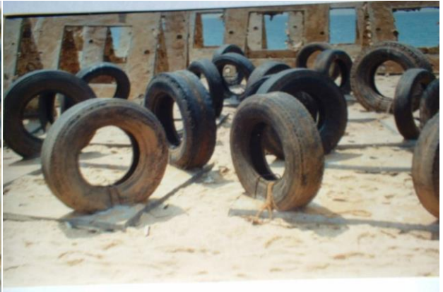
Low cost modules (Old tyres mounted on concrete slabs, Poovar, Trivandrum)
