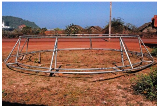
Low cost cage before epoxy coating
