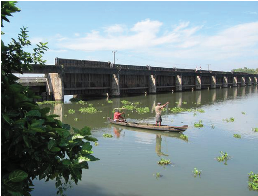
Figure 3.—The Thanneermukkom Bund (barrier), 2 km (1.25 mi) long, that divides Vembanad Lake into two sub-equal halves. A roadway for automobiles runs along its top.
