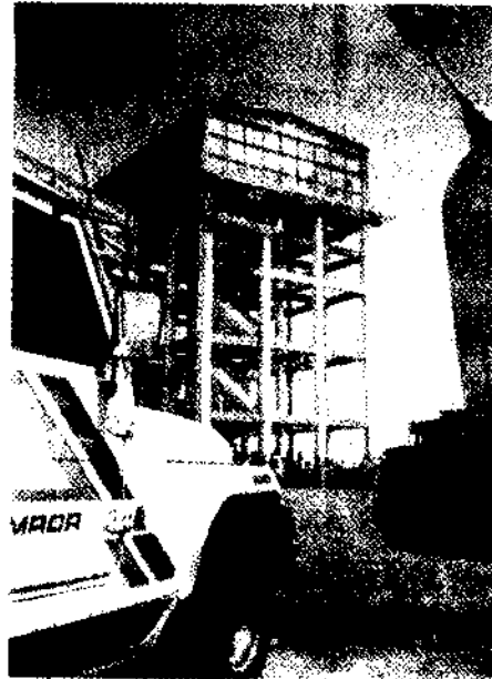
Fig. 7. Larger water tank at the new jetty of the Sassoon Docks Fisheries Harbour, Mumbai.
