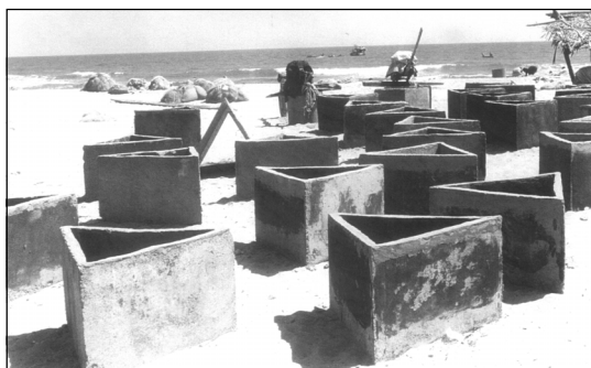
Ferrocement triangular structure
