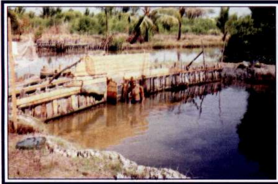
A view of a fabricated sluice
