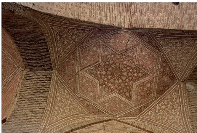
Detail of one of the vaults of the upper gallery
