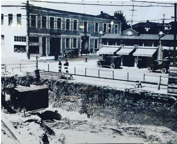
The site of the future Neptune Theatre (at the corner of 45 th Ave. NE & Brooklyn Ave) being excavated for construction in 1919. Courtesy STG Archive and Gallery.
