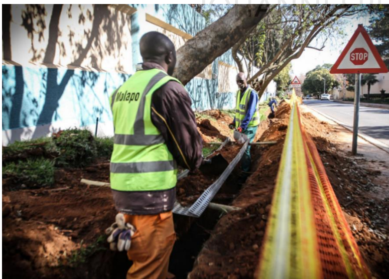
Figure 13: Installation of optic fiber lines in Sandton
