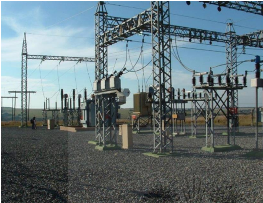
Figure 10: Battery demo facility for 2000 Mega-Watts energy storage, Rosherville
