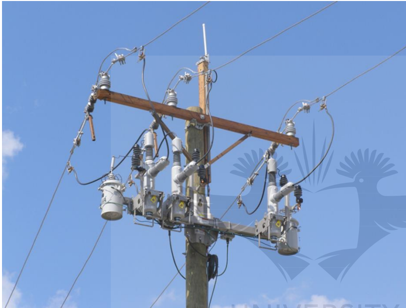
Figure 16: Solid Dielectric Triple Option Recloser, up to 38kv
