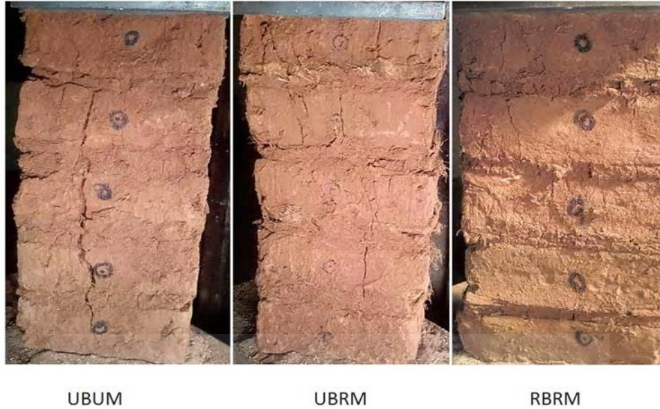
Figure 12.6 : Failure modes of masonry prisms.
