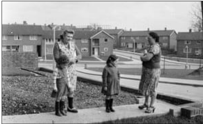
Figure 10: Council housing in the new town of Hemel Hempstead, Hertfordshire in 1954. (Photograph: Raymond Kleboe/Getty Images, Guardian Newspaper 17 July 2019).
