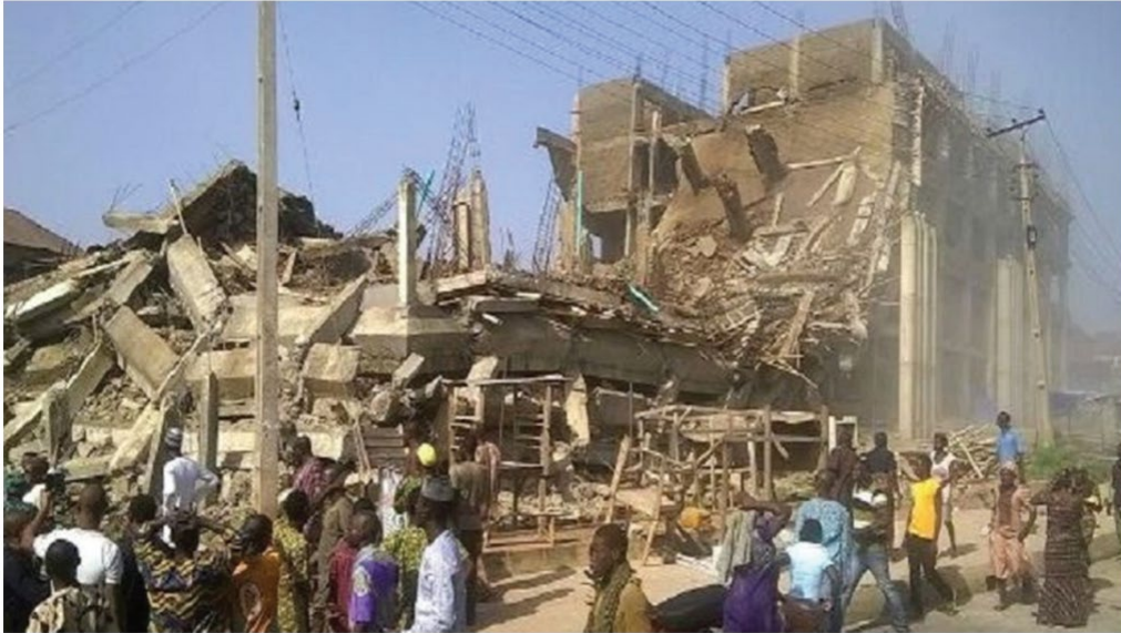
Figure 1: Meiran Building Collapse. Source [17].
