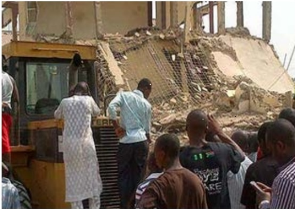
Figure 2: Clearing of debris on the Naval Building site. Source: [18].
