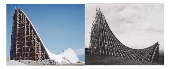
Plate 3. 13: Hyperbolic paraboloid thin-shell structure can be casted on straight surfces Source: Ressler (2017)
