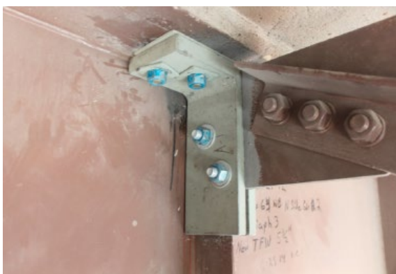
Figure 4: Repaired web-gap view (Source: [16])
