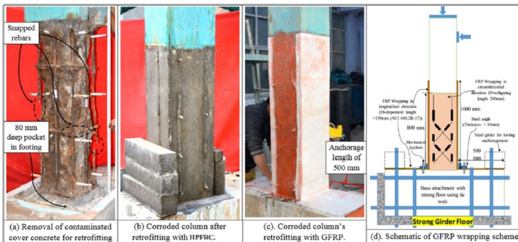
Figure 3: Retrofitting of corroded RC columns (Source: [15])
