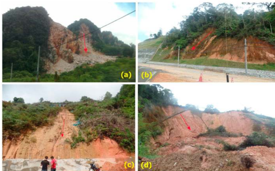
Figure 3. Field photographs of recent landslides and types of landslides: (a) a shallow translational rockslide, (b) a shallow translational slide at the road side, (c) a rotational slide and (d) deep-seated rotational slide. The arrow depicts the movement direction.
