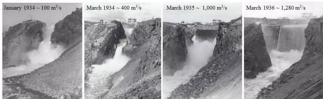
Figure 1.1. Evolution of erosion at the Ricobayo Dam spillway (Annandale, 2006).
