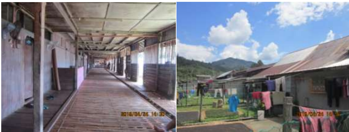
Figure 1: Left, the long gallery or awah still in traditional form. The floor made from split bamboo. Right, modernization occurs at the apartment section of the longhouse, especially in the kitchen and backyard area. Materials such bricks and concrete are used to replace timber and bamboo. Image Copyright, Victoria (2015).
