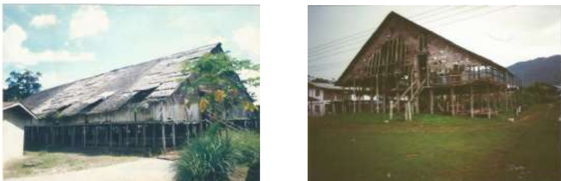
Figure 3: Bidayuh traditional longhouse of Kpg Merian Bedup, Serian. Left: Roof flap window or kamban can be seen where it functions both for natural lighting and ventilation. Timber shingles and sago thatch are used as roof coverings. The longhouse was completely demolished in the year 2011. Image Copyright, Victoria (2015).
