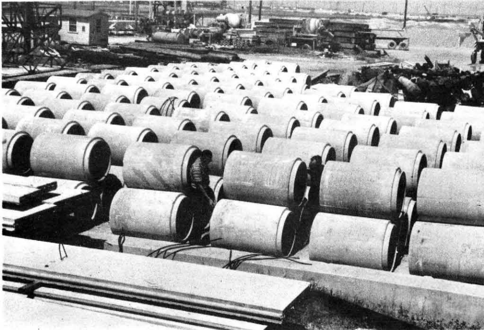
Figure 5 Assembly of pipes for Unit No. 4 of Galveston Reef.
