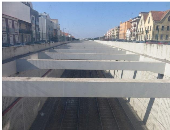
Figure 1 – Railway line along a trench: Espinho, Portugal
