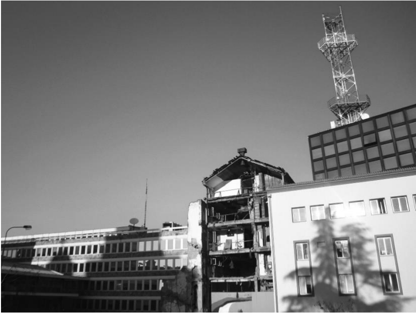
Figure 5.3 The unreconstructed section of the Radio Television of Serbia (RTS) building.
