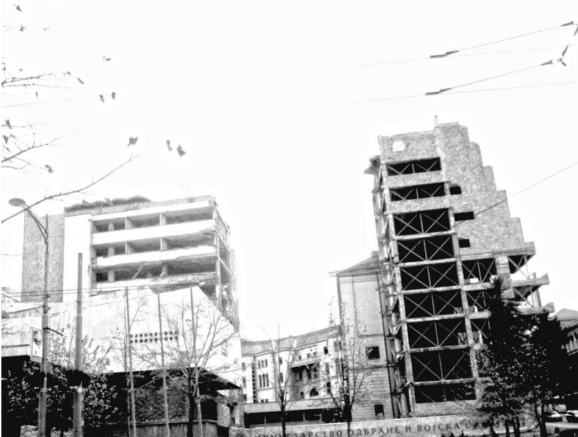
Figure 4.3 The Military Headquarters (Building A) in 2014 and in 2017.
