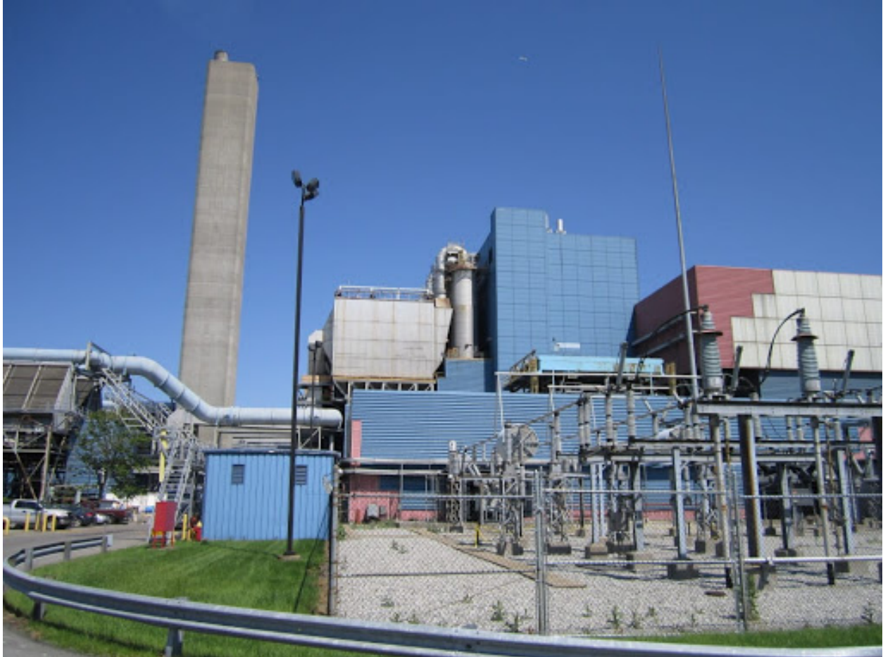
Figure 13. The Essex County Resource Recovery Facility in New Jersey. 2012. http://www.lseacorp.com/portfolio/pany.html . Copyright 2012 by the LS Engineering Associations Corporation.
