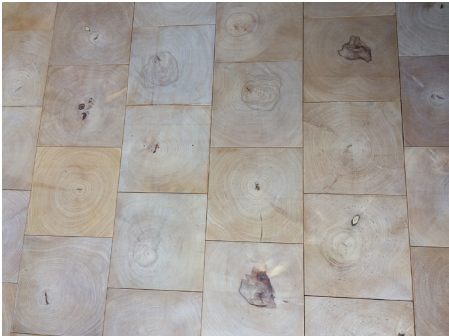
Figure 4: An example of a flooring commission recently completed by Kenton Jones Ltd. using end grain birch tiles.
