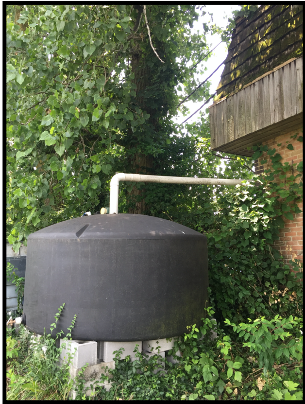
Rainwater collection in Garden B
