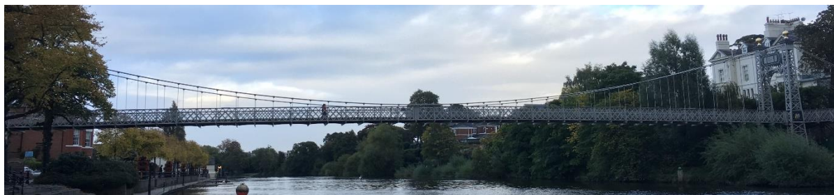
(a) Overall view of Queen's park footbridge
