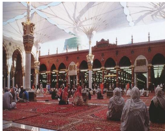
Figure 1: The Inner courtyard of the Mosque of Madinah showing its shading system [6].
