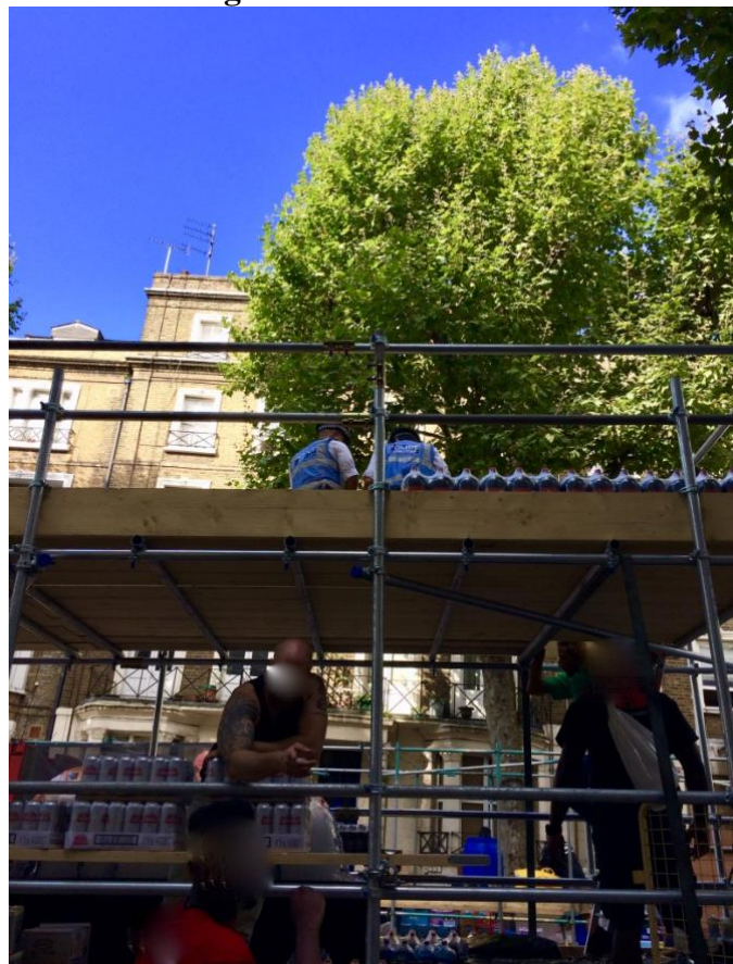
Image 22: Float construction and PLT
