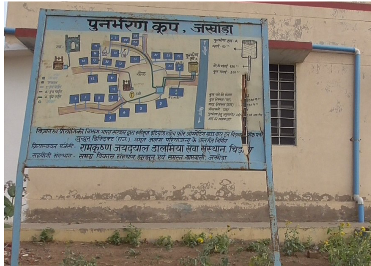
Figure 2. The rainwater harvesting system in Jhakhoda. The map shows how each house is connected to a centralised system which diverts water to recharging the aquifer after individual tanks are full.
