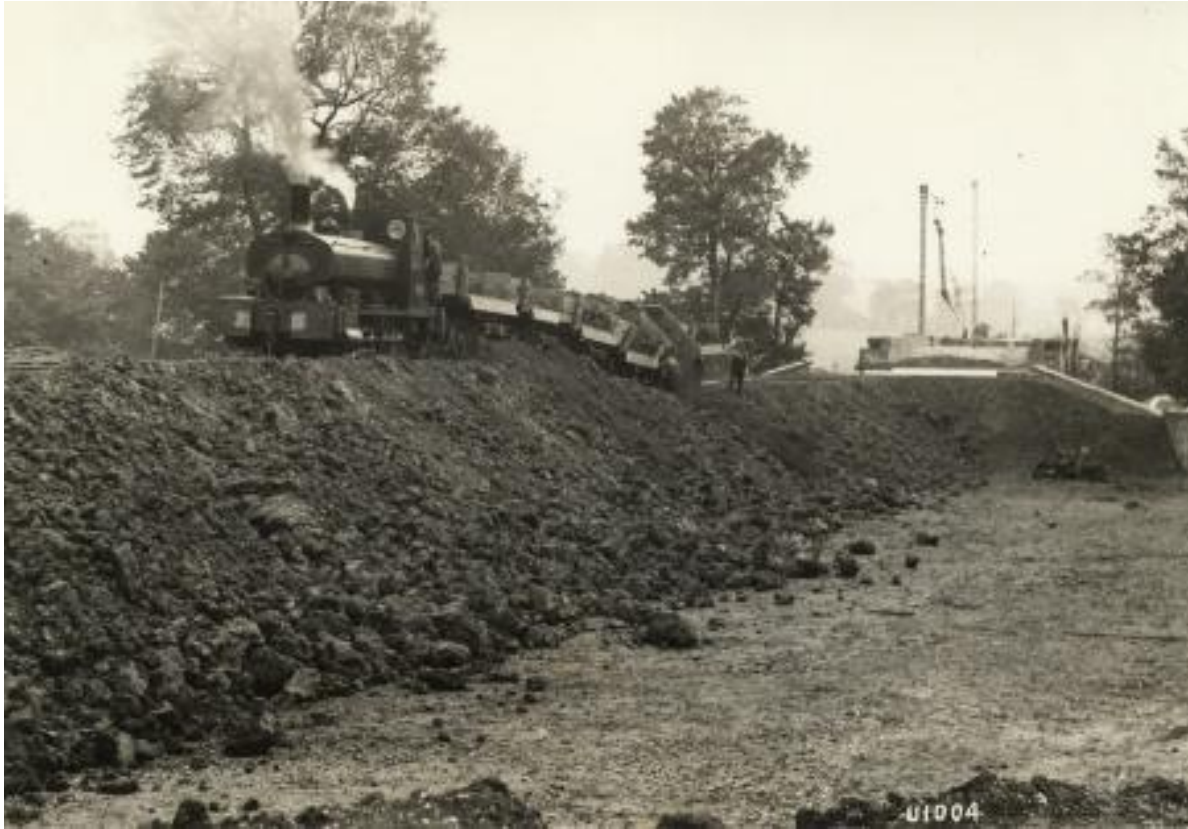
Figure 1. Formation of embankments from London Clay fill by side-tipping from railway carriages (photograph courtesy of the Transport Museum: site of Hendon Central Underground station, Northern line by Topical Press, 03/10/1922).
