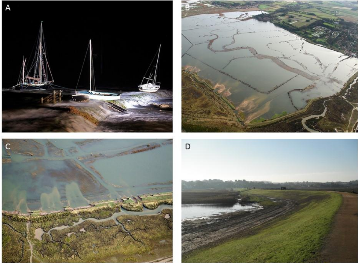
934 Figure 2: Storm surge flooding, and subsequent embankment repair, at Blakeney Freshes. A) 935 Floodwaters overtopping the southwest corner of the Freshes embankment, evening of 5 936 December 2013 (photo: © Stuart Warrington); B) Post-surge flood extent, 9 December 937 2013. Note extensive alluvial spreads into the Freshes from major bank failures along 938 northern boundary (aerial photography: M Page ( http://mike-page.co.uk/ )); C) detail of 939 breaches on northwestern boundary (aerial photography: M Page ( http://mike- 940 page.co.uk/ )); D) repaired and re-profiled embankment, southwestern section (photo: T. 941 Spencer 30.12.2014).
