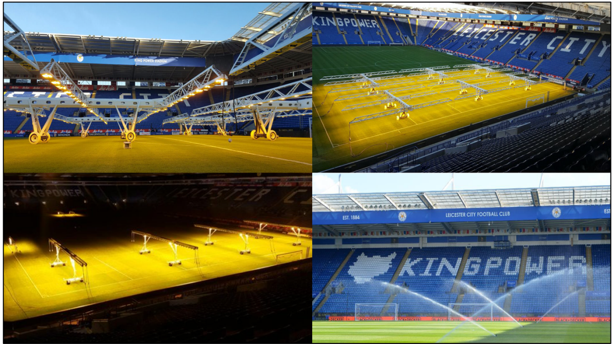
Figure 2.3 Advancing technology such as pop up irrigation sprinklers and artificial growing light ensure year round growth of the natural turf pitch.
