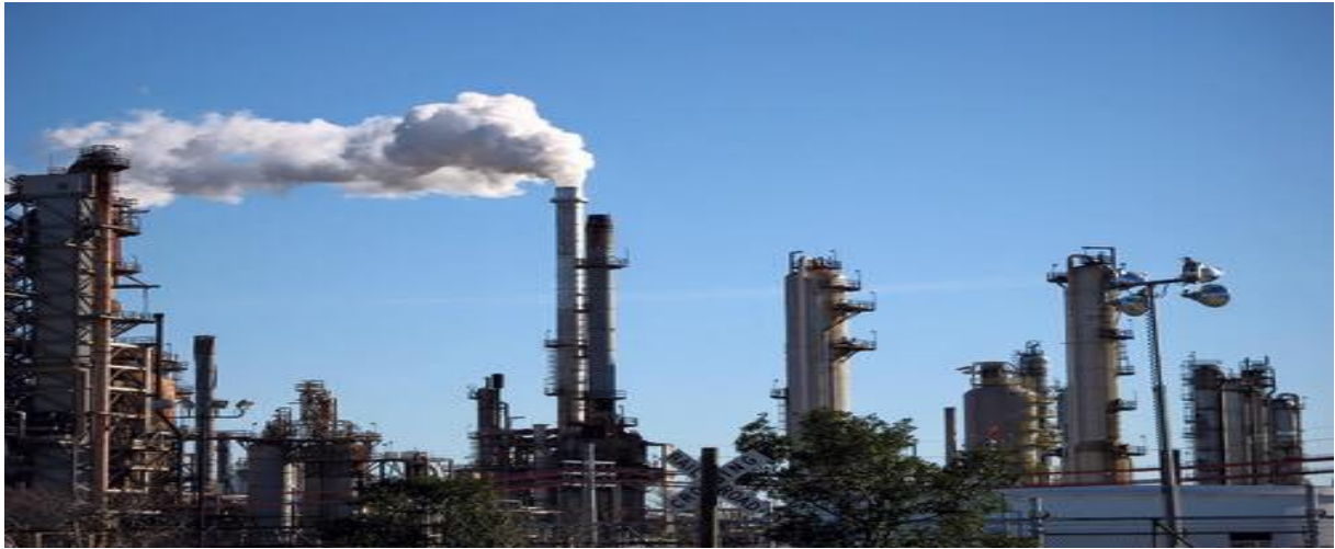
Figure 8.1: The picture of Kaduna Refining and Petrochemical Company Limited (KRPC)
