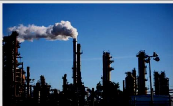
Figure 1: The picture of Kaduna Refining and Petrochemical Company Limited (KRPC).
