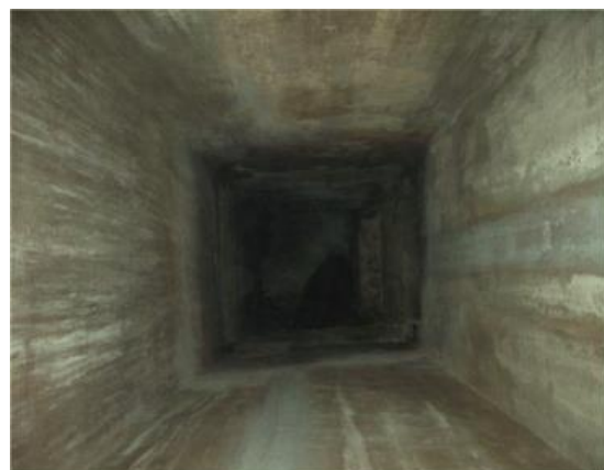
(b) Shaft after repair in 2009
