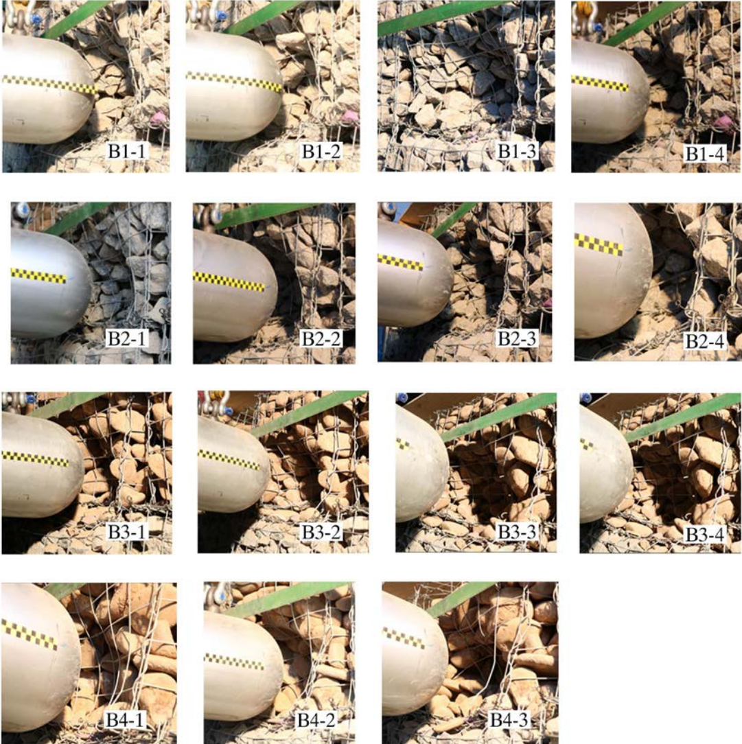
Figure 4.42 Damage to the gabion cushion following the impact – Test Series B
