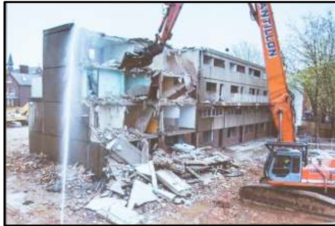
Figure 4.3: Demolitions for luxury apartments in London
