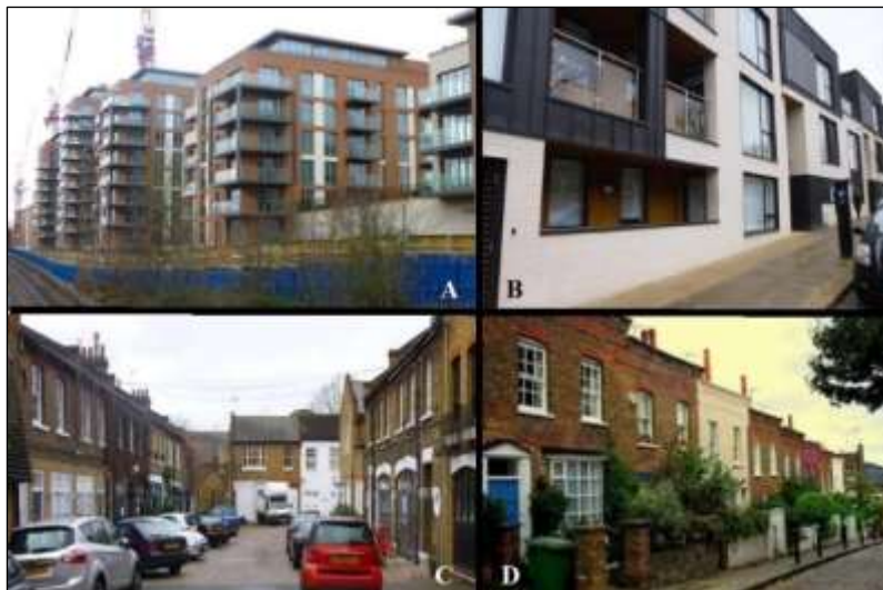
Figure 4.2: The modern (A, B) and the traditional (C, D): Affordable and rental housing in Willesden, London
