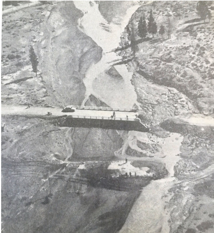
Figure 58: A bridge destroyed by the Loxton floodwater. Source: Die Burger, 29 March 1961, p.1.
