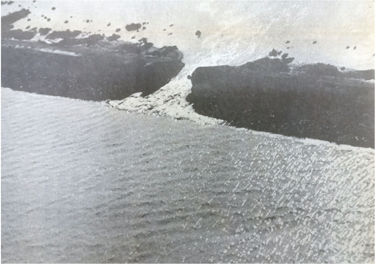
Figure 59: The collapse of Loxton dam wall. Source: Die Burger, 29 March 1961, p.9.
