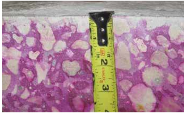
Fig. 6. Measurement of depth of carbonation.
