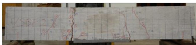
Figure 6. Crack pattern of VSSB
