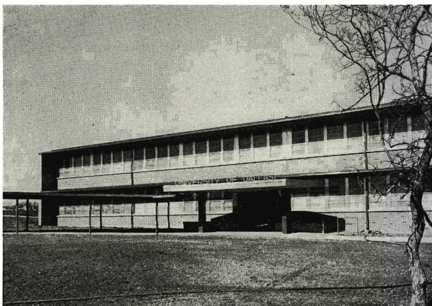
Main entrance to the Science Building. The covered walkway at left connects with the Lecture Hall.
