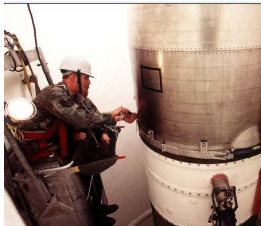
Figure 19: Technicians Working from Elevator Workcage (LGM 30 Minuteman III)
