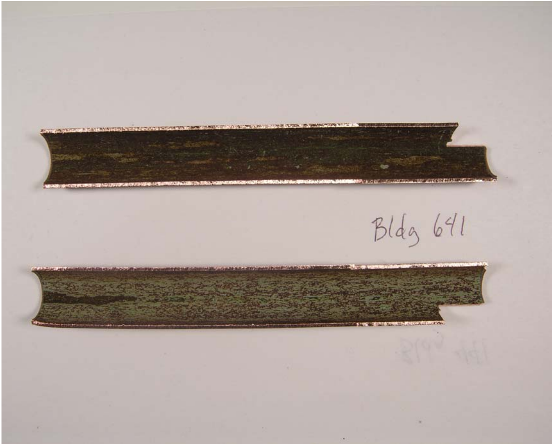
Figure G.16. Digital picture of the copper pipe.
