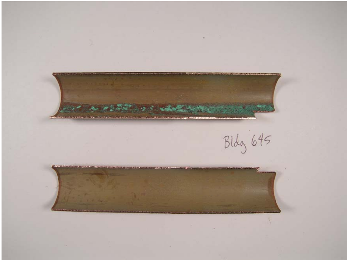
Figure G.59. Digital picture of the copper pipe.
