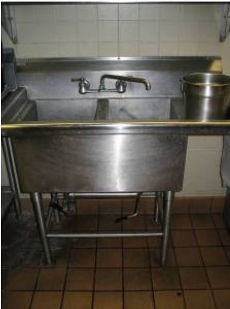
AAFES kitchen sink. Sample taken from under the sink
