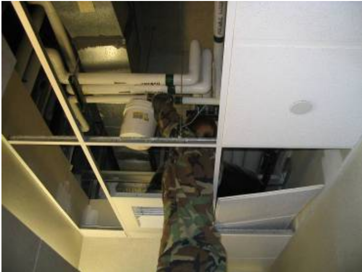
Sampling above the ceiling above the kitchenette sink.
