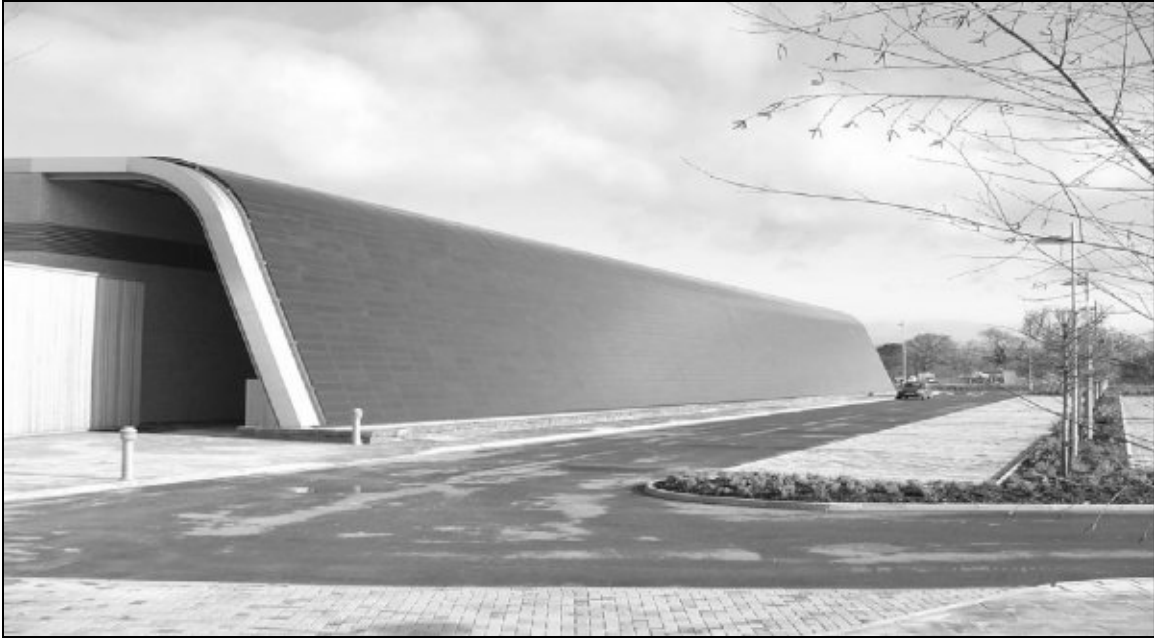
Figure 8: An Application of CIGS (Zweibel, 2004). CIGS used in a building-integrated form.
