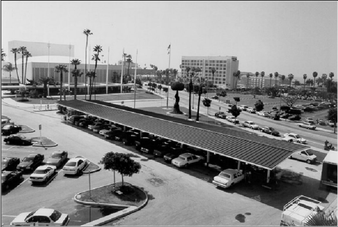
Figure 10: An Application of a-Si (Zweibel, 2004). A covered parking area decked with a-Si modules.
