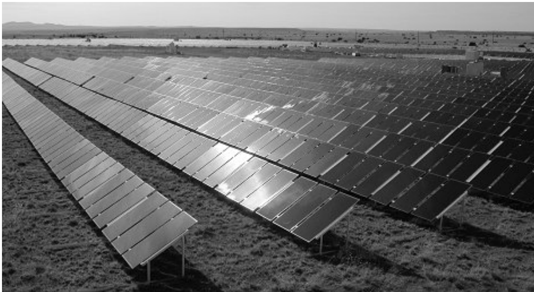
Figure 6: An Application of CdTe (Zweibel, 2004). A CdTe field array.
