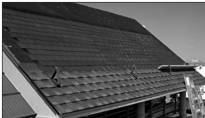
Figure 11: Photovoltaic Shingles (Oksolar.com, ND). Photovoltaic shingles (the darker shingles) appear very similar to conventional shingles and perform equally. Installation of photovoltaic shingles actually precludes the use of other roofing materials.
