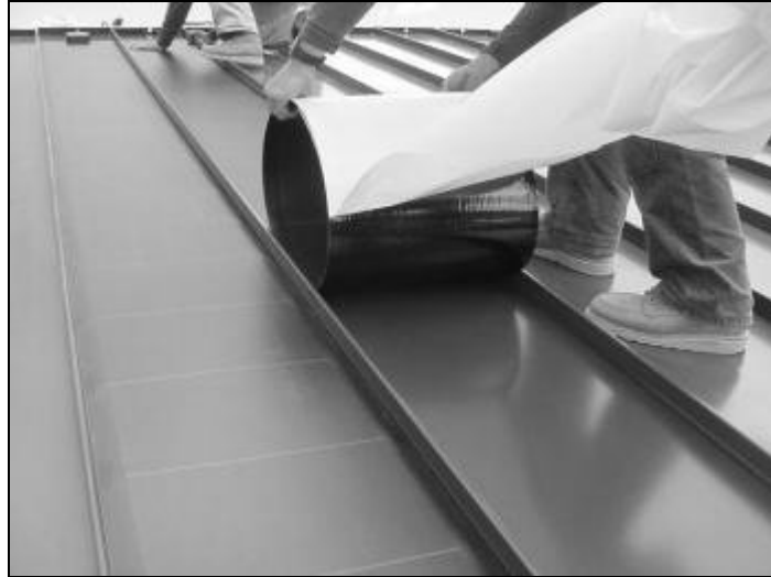
Figure 12: Photovoltaic Rolls (JRCCI Products and Services, ND). Photovoltaic cells on a flexible substrate are delivered in rolls which can be glued between the seams of a standing seam metal roof. This photo shows the backing being peeled off of a flexible roll exposing the adhesive surface.
