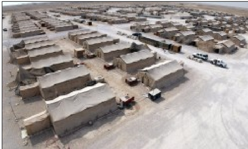
Figure 1.1. Prepositioned Assets. TEMPER Tents are commonly used for initial beddown of forces (Global Security, 2005a).
