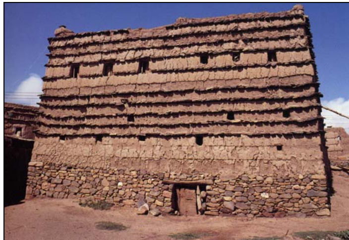
Figure 2.21. Drip Edges. Slate projected from walls to direct water away from the façade (King, 1998).
