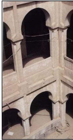
Figure 2.19. Protective Plaster Coating. Sandstone walls were rendered smooth with a protective plaster coating (King, 1998).
