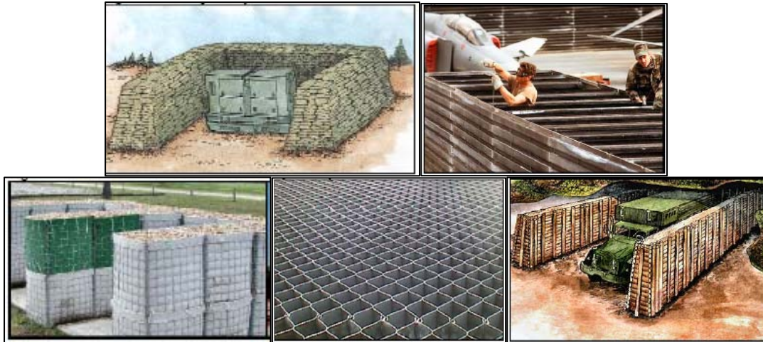
Figure 2.3. Revetment Materials. Common revetment materials include (a) sandbags, (b) metal panels, (c) fabric containers, (d) grids, and (e) logs (AFP 10-219, Vol. 7, 2004).
