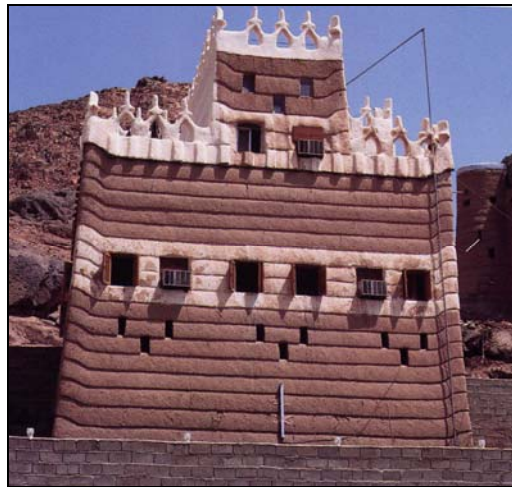
Figure 2.22. Unique Regional Style. Modifications to control erosion and earthquake damage produced a unique style in Najran (King, 1998).
