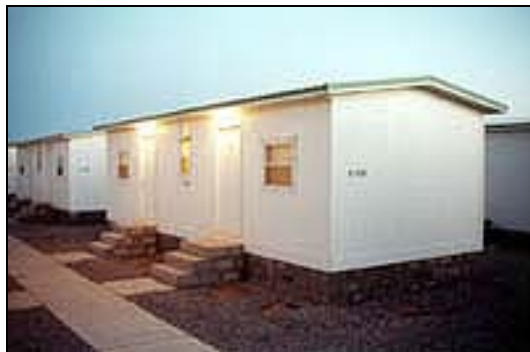
Figure 2.7. Prefabricated Metal Buildings. Prefabricated metal buildings are a popular permanent construction method (RED SEA Housing Services, 2005).
