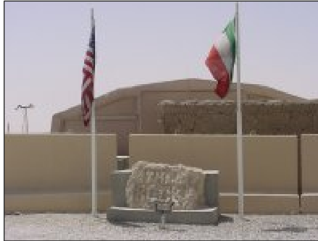
Figure 1.3. Barriers. Concrete barriers are a common blast mitigation measure (Global Security, 2005c).
